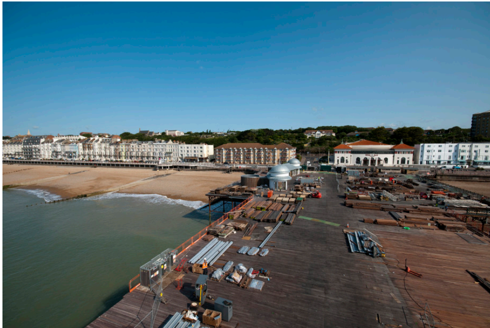
An aerial image of Hastings Pier during the reconstruction in 2015 (HPC100.035)
